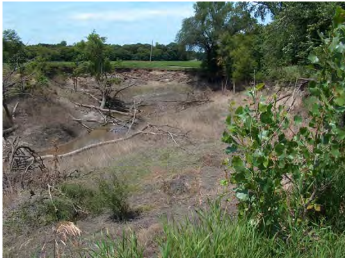
Photo E – Existing Cutoff Ditch Bank Failures
